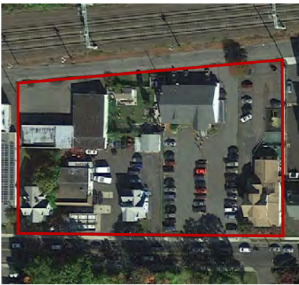
2. New Haven Avenue: Several adjoining parcels on New Haven Road and Buckingham Avenue (106, 112, 124, 132 New Haven Road and 57 Buckingham Avenue) are currently comprised of low density land uses such as a gas station, single family residence, Elks club, and day care. If assembled, these parcels would comprise a 1.95 acre site within walking distance of the train station.
