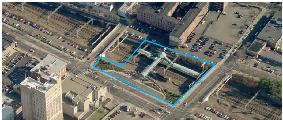
Birdseye view of State Street Station site. Source: Bing Maps
